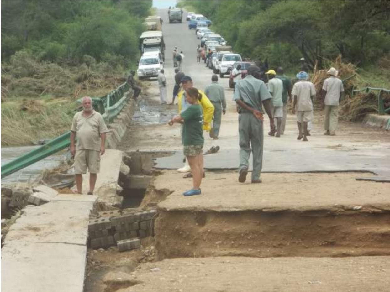
Bridge in Kruger Park damaged by rain water
